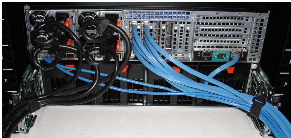
Figure 8. Cable routing without a CMA
