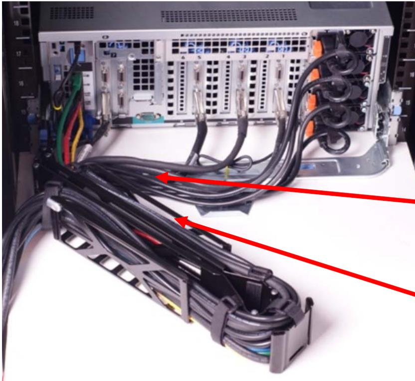
**NOTE:** Do not store excess cable slack inside the CMA. The cable may protrude through the CMA, thus causing binding and potentially damaging the cable.
