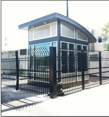
Fresh Air HotHouse
